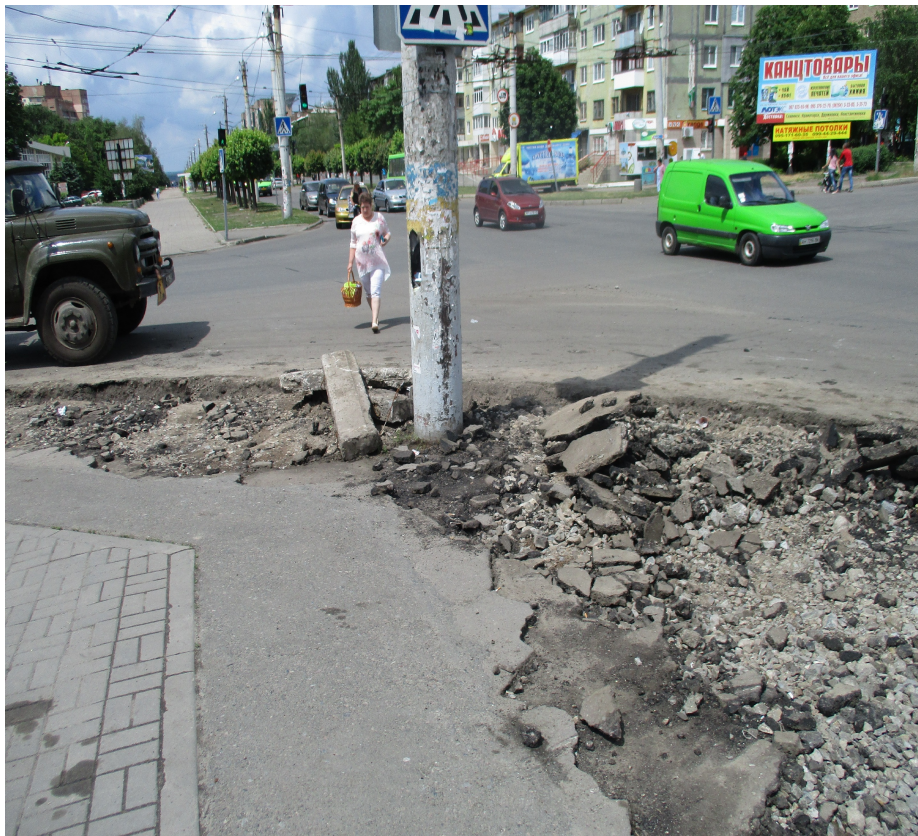
Street construction. No barricades or yellow tape people walking right through the middle of all this.
